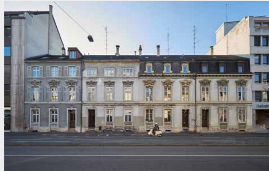
The houses at Steinengraben have been in discord with their owners for a long time: the Helvetia Insurance company wants to tear them down and create an office building.
